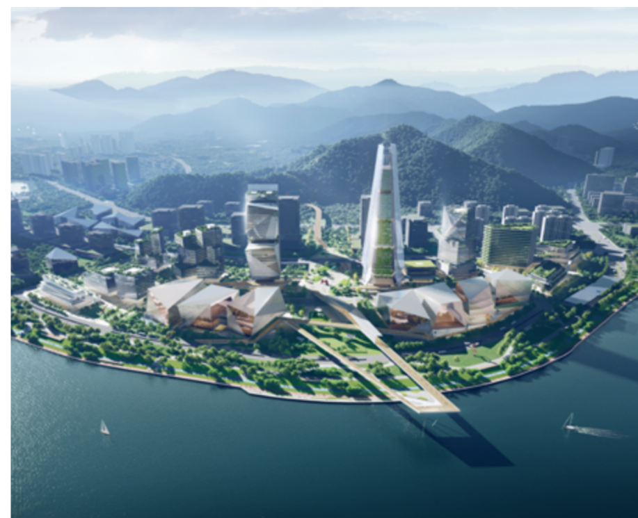
临安城市客厅/LinAn City Lobby Hangzhou - China
